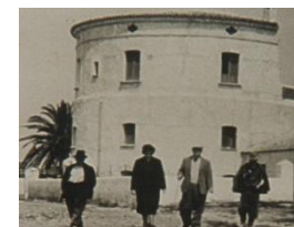
Torre Bollitta a Nova Siri
